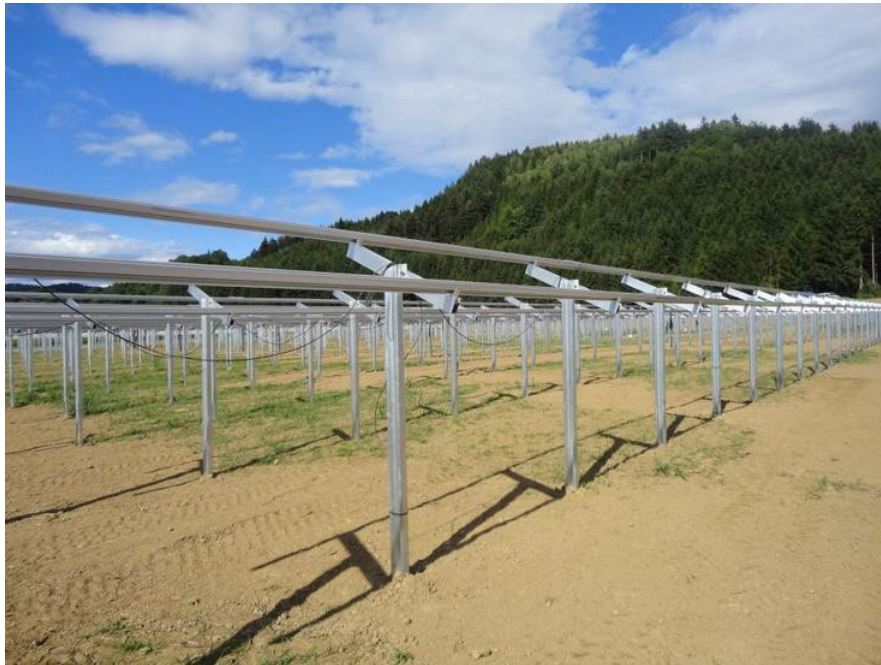
Racking equipment – prior to panel installation.
