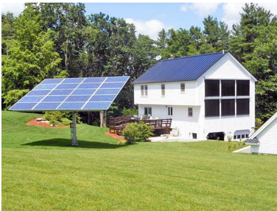
Tracker Mounted Residential System: Courtesy Revision Energy
