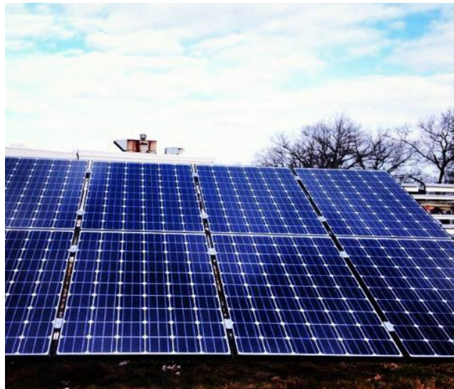
Completed installation showing gaps between panels
